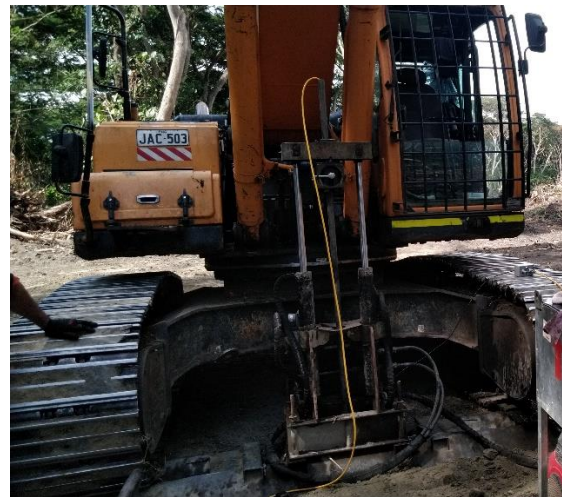
Figure 4. Portable in-situ testing rig supported by excavator
